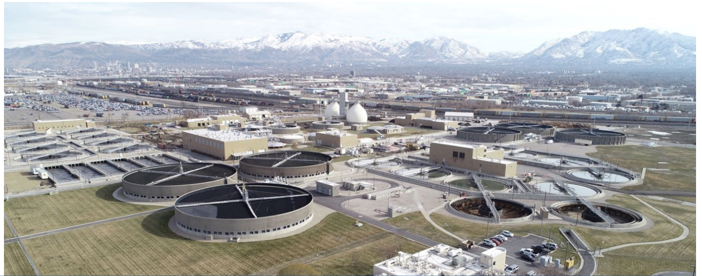
Utah Lake Water Reclamation Facility Upgrades
